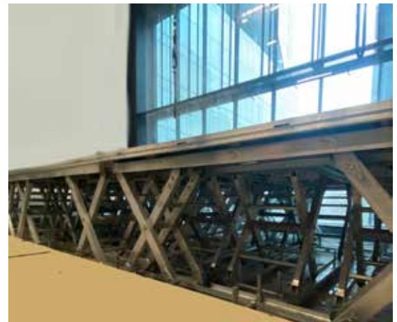
SHOWLIFT DURING INSTALLATION AT MASSEY HALL
